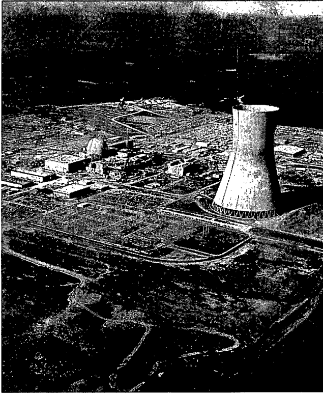
In early January 1987, the NRC authorized the issuance of a full-power license for the Shearon Harris nuclear power plant (shown here during construction), near New Hill, N.C. In August 1987, the United States Court of Appeals for the Fourth Circuit upheld the Commission decision and rejected an intervenor petition regarding emergency planning for the facility.
