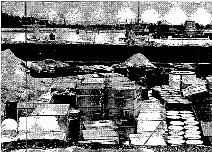
This is a low-level nuclear waste disposal site at Barnwell, S.C. The trench is nearly full and will soon be covered and sealed.
